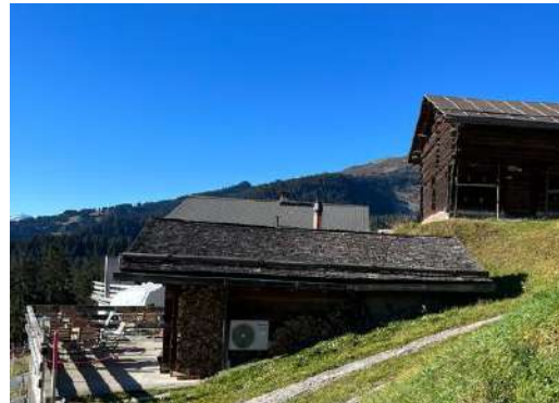
Alpine restaurant, Flims, 4 kW
