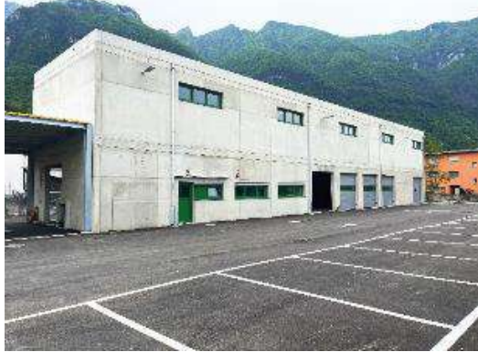
Commercial building, Melano, 13 kW
