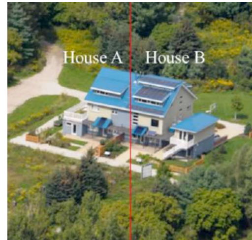
Archetype Sustainable House (ASH) Twin Houses of the Toronto and Region Conservation Authority (TRCA)
